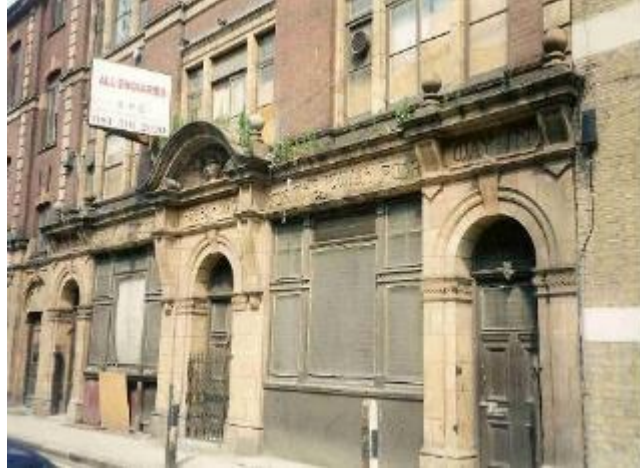
Figure 11a-c: Photographs showing the gentrification of the former Jewish Soup Kitchen on Brune Street, E1, built 1902 closed in 1992
